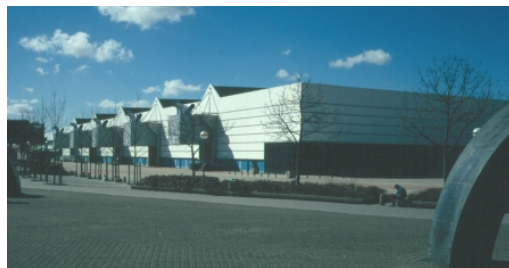
Prins-van-Oranje-Hall, Utrecht fair, ATES for cooling and for pre-heating of ventilation air
