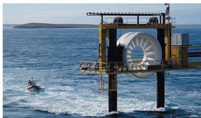
Fig. 5 – The OpenHydro tidal energy system
