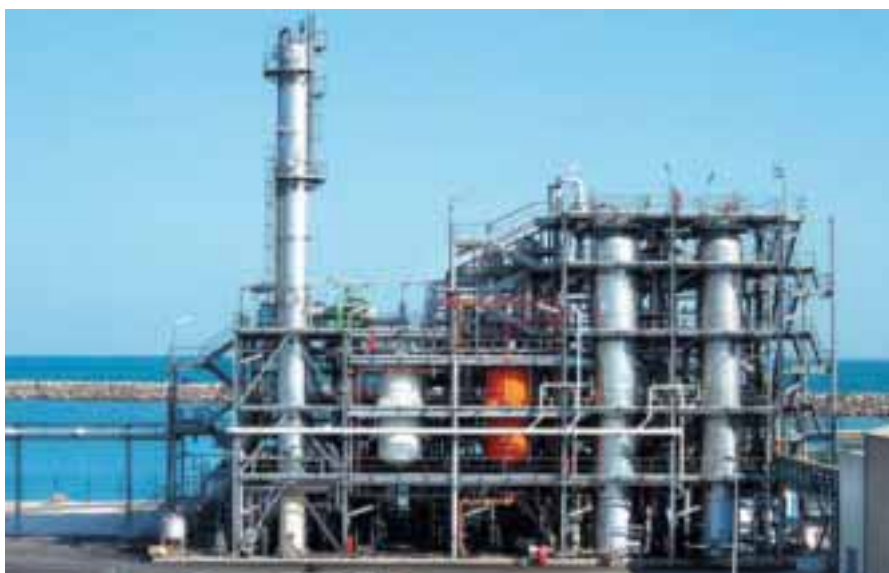
Diester Industrie's biodiesel production unit in Sète (France) using Axens' Esterfip-H™ technology.
