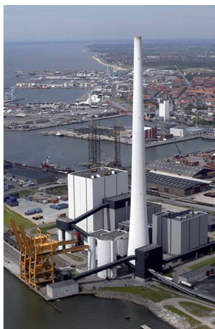
The world's first industrial pilot unit was installed in the Danish Dong Energy power station in Esbjerg as a part of the Castor project in 2006.
